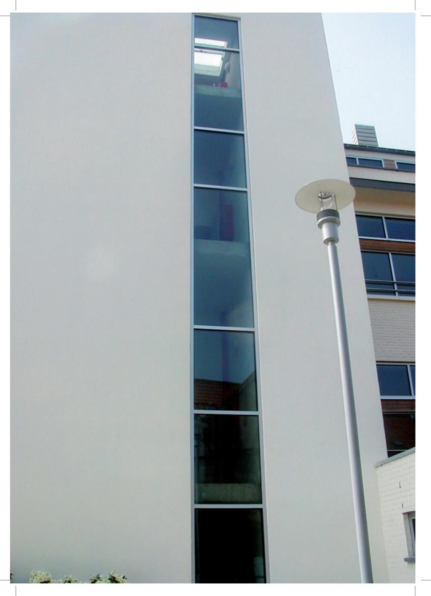
Excellence 95 HV is high performance thermally broken four chamber system with a building depth of 95mm. The system is designed to meet the increasing demands of large surfaces and ribbon windows with high stability and thermal performances with a minimal sightline.
