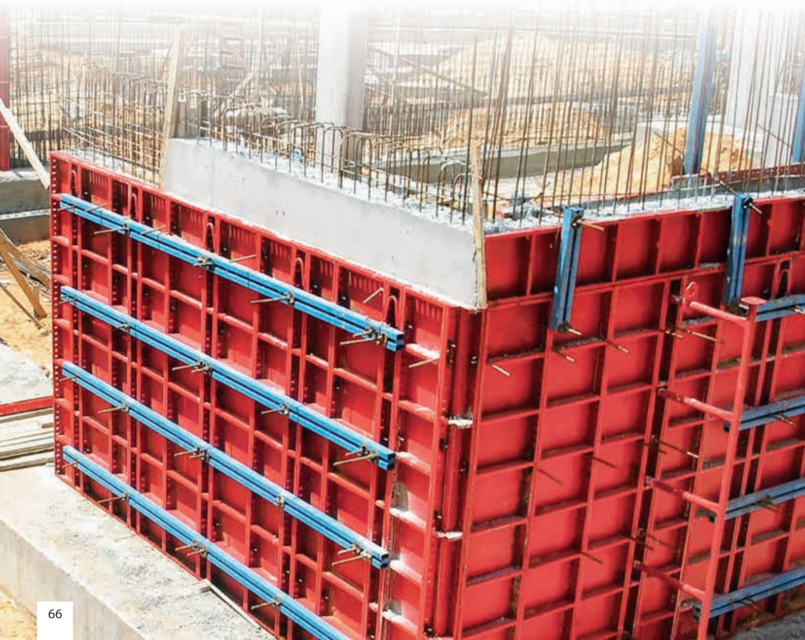
Pimli Kalıp / Formwork with Pin
