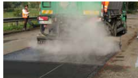
Apply bitumen emulsion
